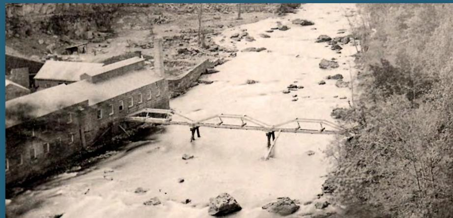
The Passaic Water Company's first pump house of the 1850s was in a complex of mills below the Great Falls, later redeveloped as the Allied Textile Printers (ATP) Site. Water was pumped across the "broomstick" bridge, shown here in a photograph of about 1870. The bridge's pipe sent water to a reservoir in the area of Hinchliffe Stadium, directly behind you. Image Credit: Paterson Historic Preservation Commission.
